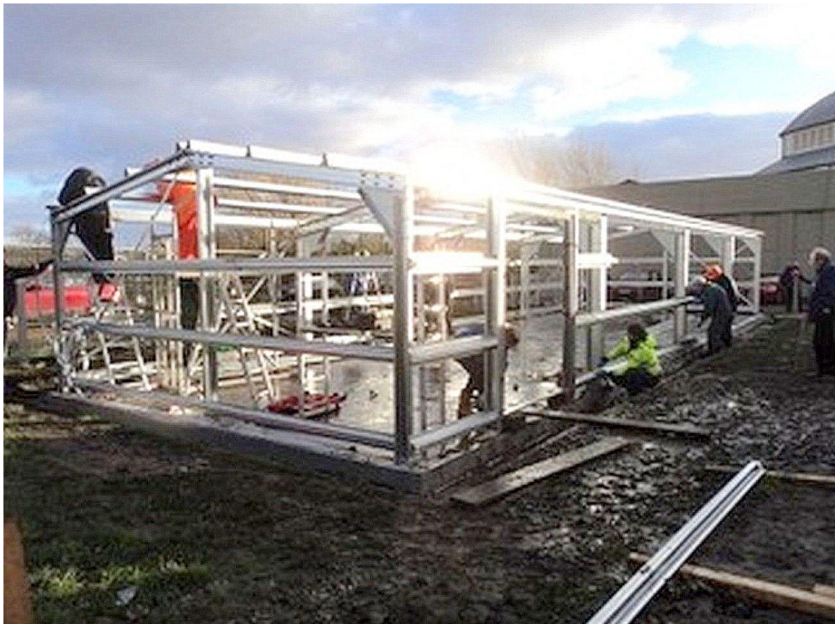
Erecting the framework. Note the mud !!!
