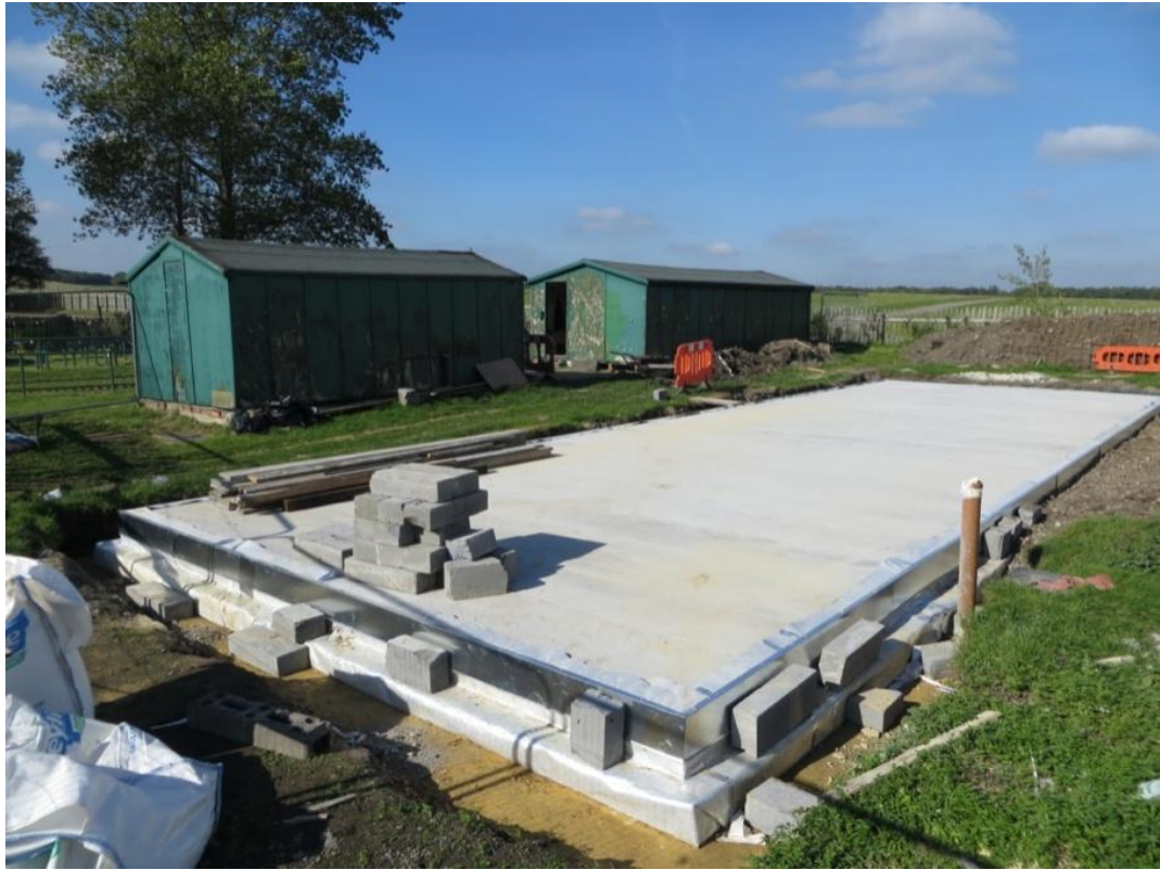
The finished floor-slab
