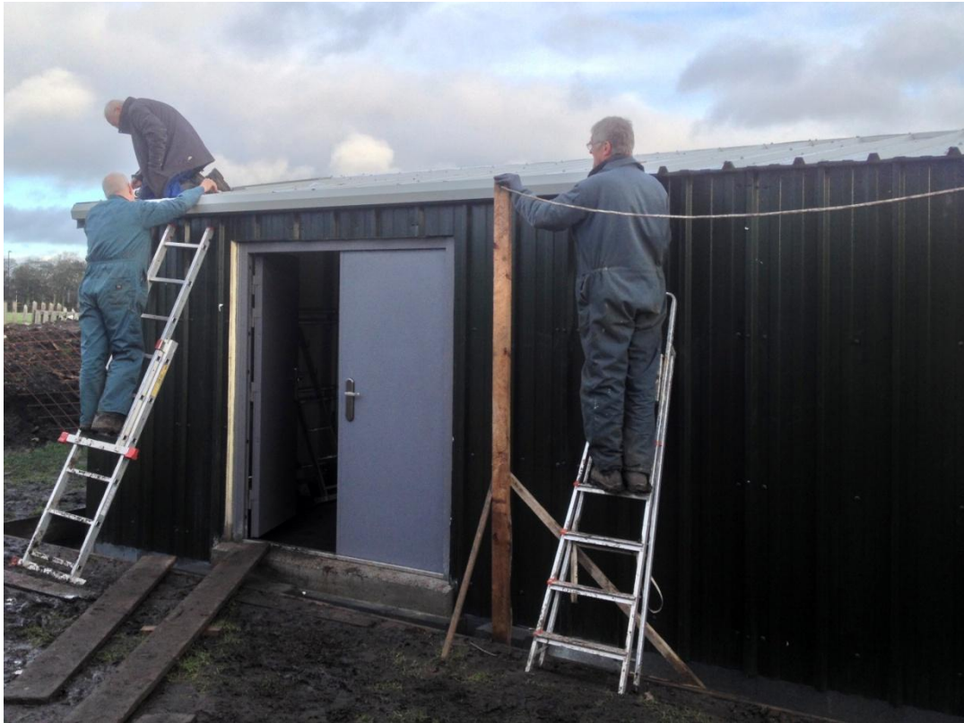
Getting close – hanging the guttering
