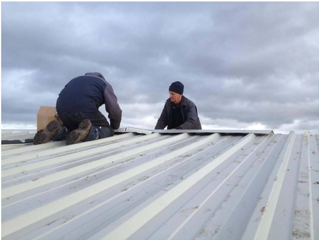
Laying the roof
