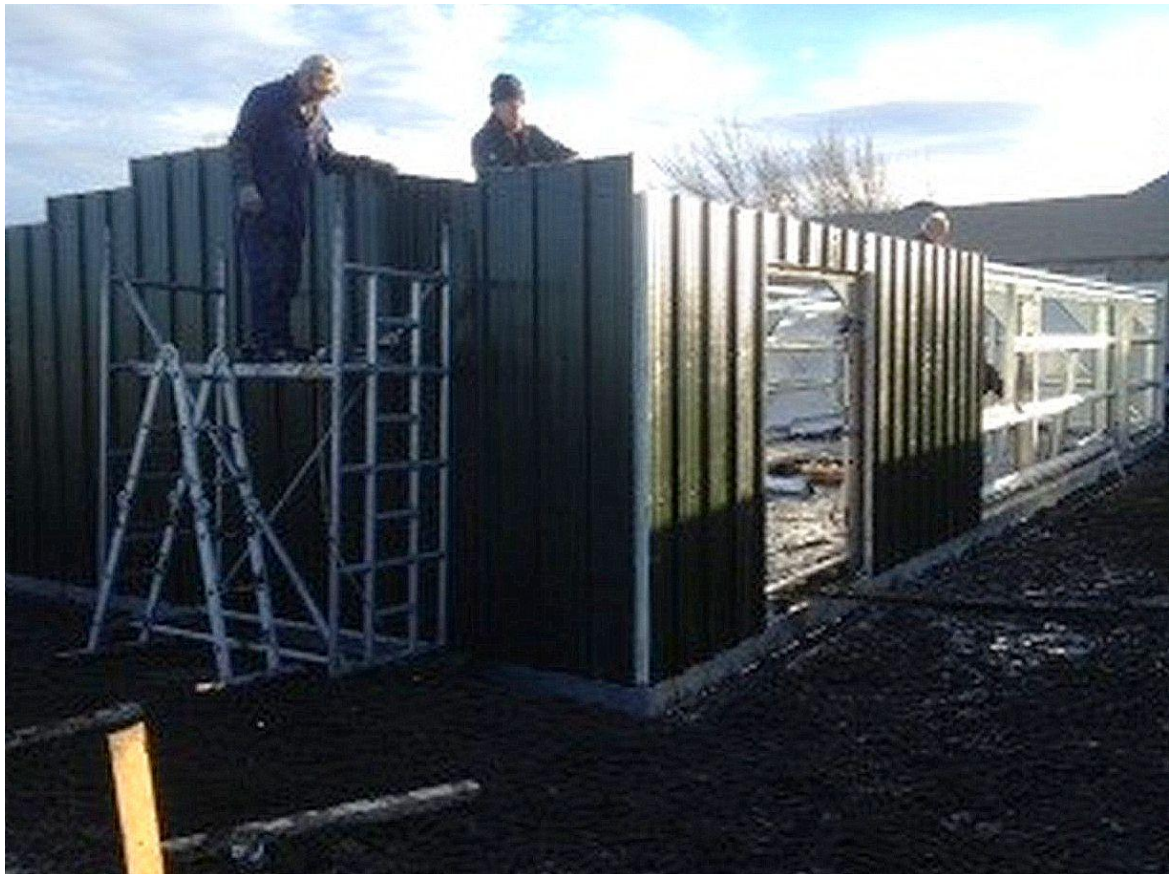
Fitting the external cladding
